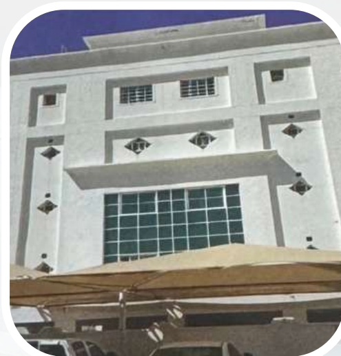
Residential building (Al Khuwair) We maintained the alarm system, extinguishers and fire pumps
