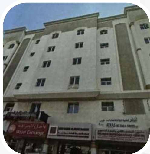
Commercial Building (Azaiba) We performed maintenance for fire alarm systems, fire extinguisher and fire pumps
