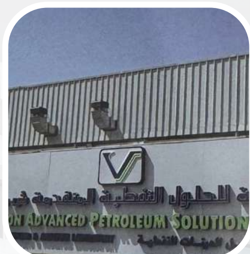
Vision Advanced Oil Solutions installed a new fire alarm system and fire extinguisher
