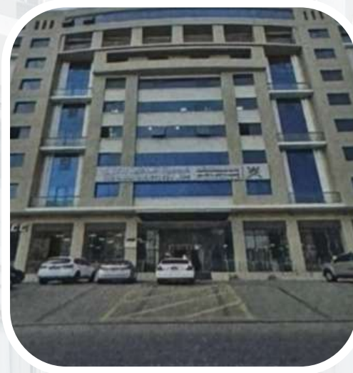
Commercial building (Ghala) We have implemented a one-year periodic maintenance contract for the fire alarm system and fire fighting system
