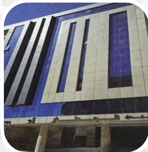
Muscat International Airport Hotel (Ghala) We installed new fire alarm systems, fire fighting systems, fire extinguishers, and fire pumps
