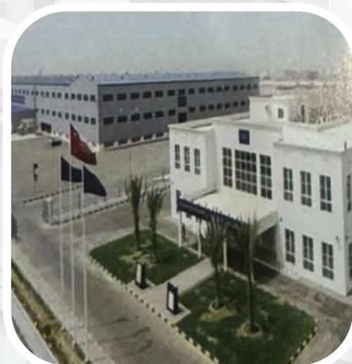
Gulf International Pipe Manufacturing Factory Manufacturing Company Maintenance of fire fighting system and fire extinguishers
