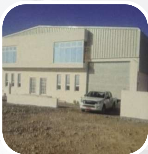
Barka warehouses Installation of alarm and fire-fighting systems and electrical works
